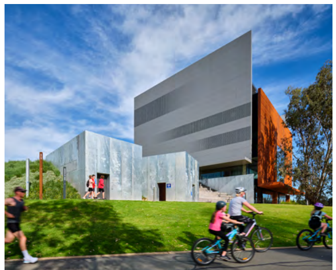
Image: The new Shepparton Art Museum, designed by Denton Corker Marshall architects, 2021. Photo: Tim Griffith.
